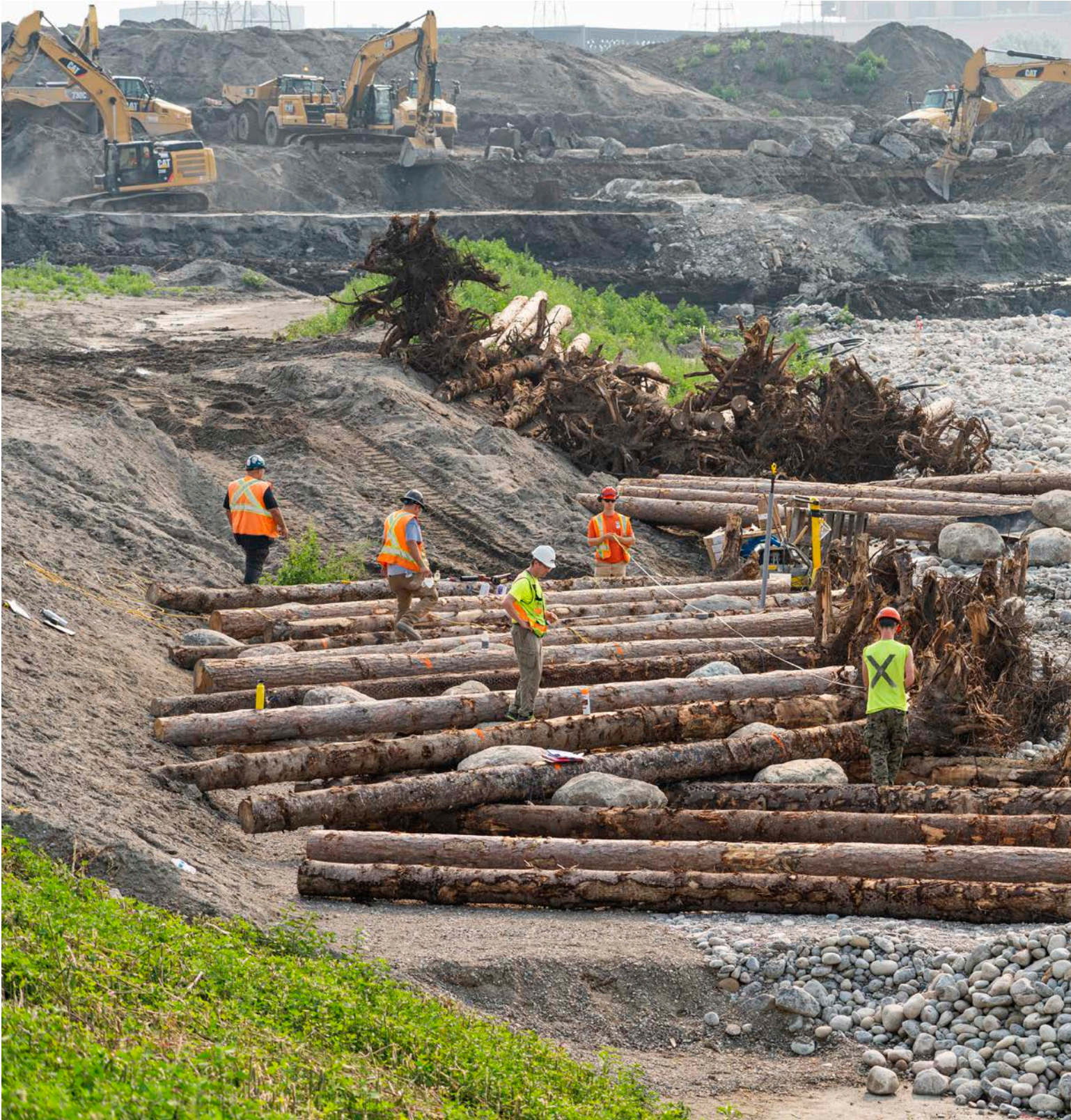
Workers place logs and rocks that will stabilize the banks of a new river valley being created in the Port Lands. See page 22 for more information and an aerial view. Image by Vid Ingelevics and Ryan Walker.
