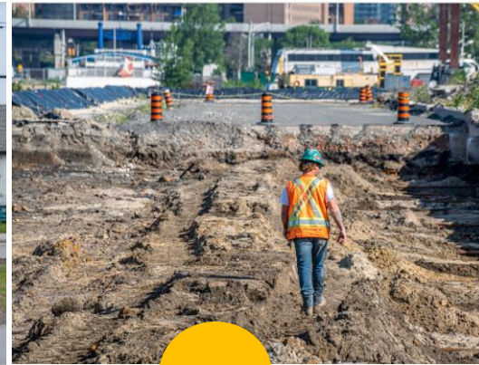
Image: Ongoing road work in the Port Lands
