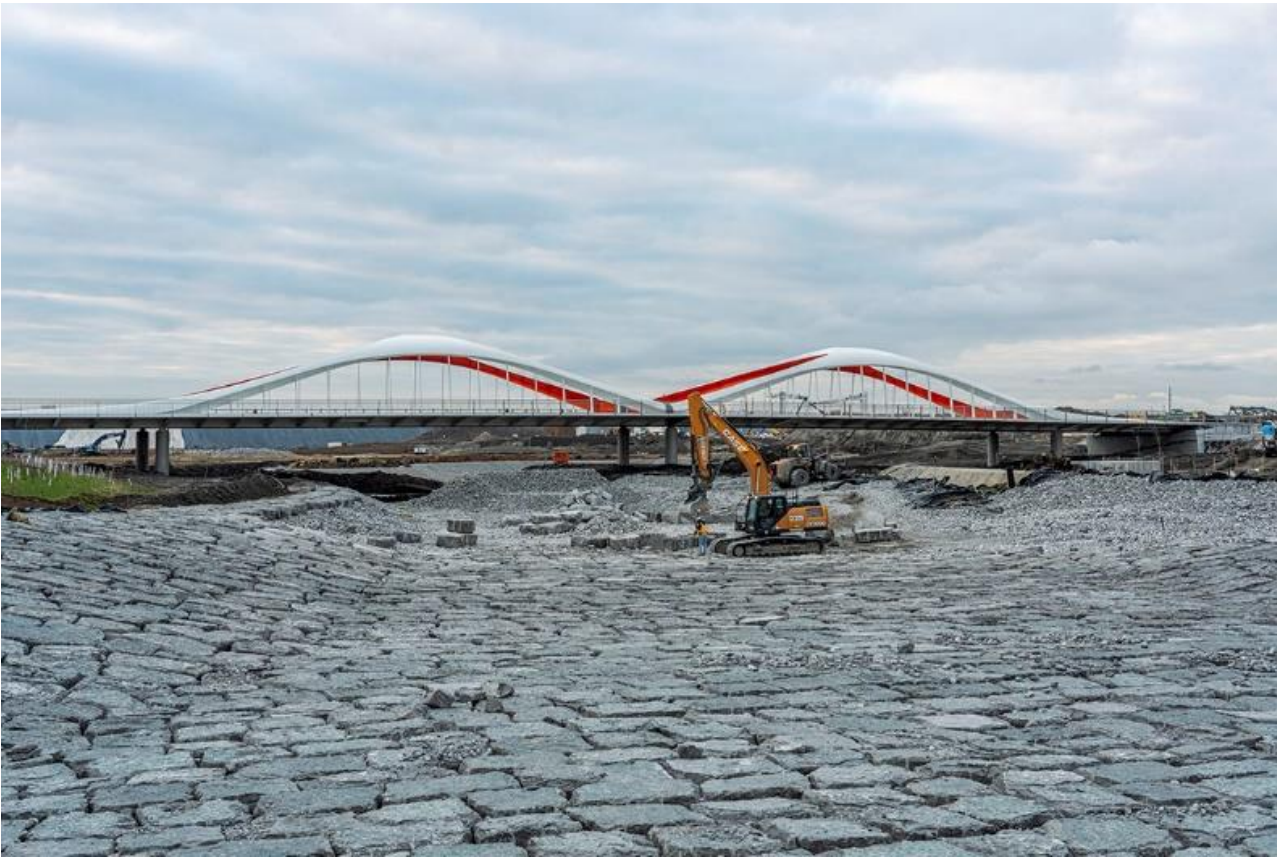
Above: The Ice Management Area, where the Don River will meet the new river valley is lined with armour stone.
