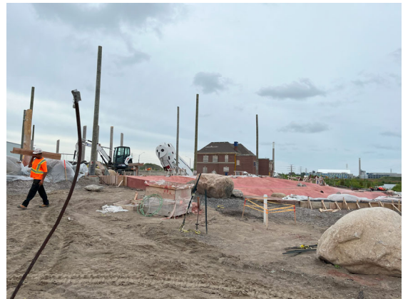
Playground – Snowy Owl works ongoing ;
