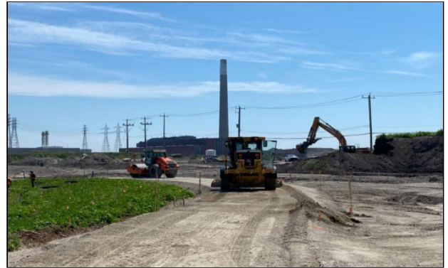
Figure 6 River Park South – Granular Placement
