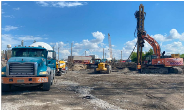
Figure 1 Don Roadway North – Final Rigid Inclusion Works
