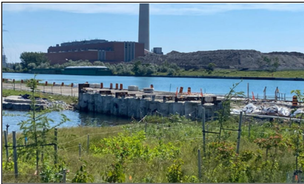
Figure 5 River Valley – South Plug Progress
