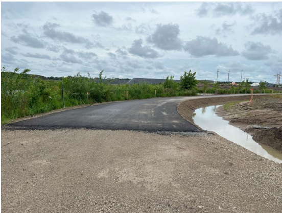
Bike Trail. – Paving works in progress;
