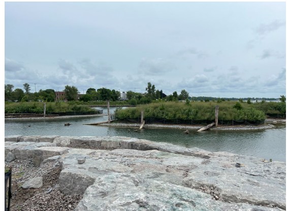
Canoe Cove. – Armour stone placement;
