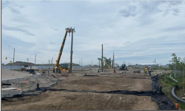
Figure 3 River Park North – Light Pole Installations
