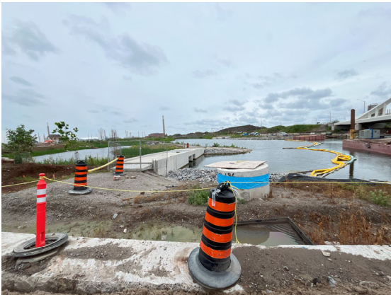
River Valley – Carp Gate settlement fixing in progress;
