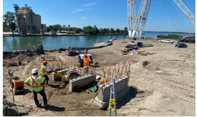
Figure 4 Canoe Cove – Staircase Footings Poured
