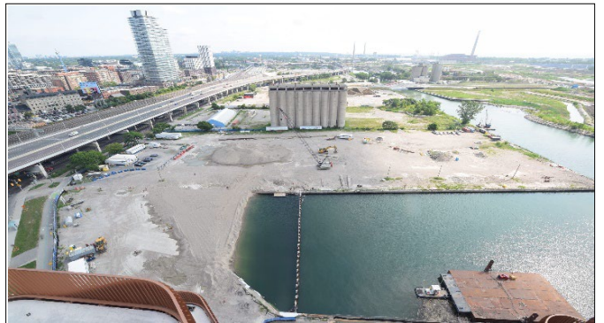
Figure 4 Parliament Lake Fill construction progress
