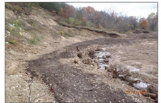
Image: Post-construction channel fill with large wood stabilization (pre-vegetation)
