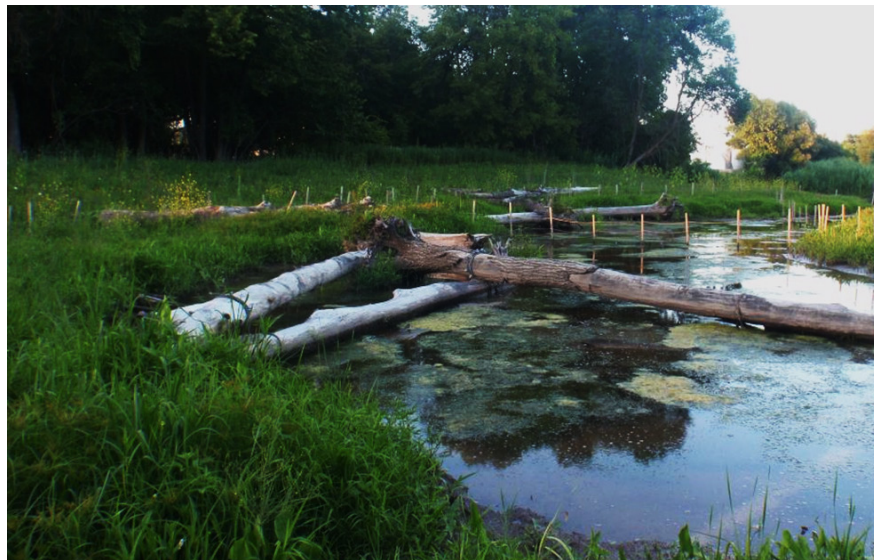
FIGURE 3-5: Examples of large wood stabilization
