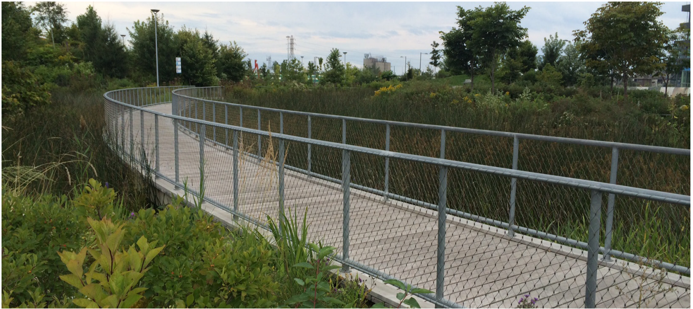
FIGURE 4-5: Example of boardwalk crossing at wetland and river channel
