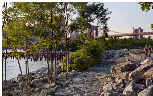
FIGURE 3-4: Armouring integrated with circulation
