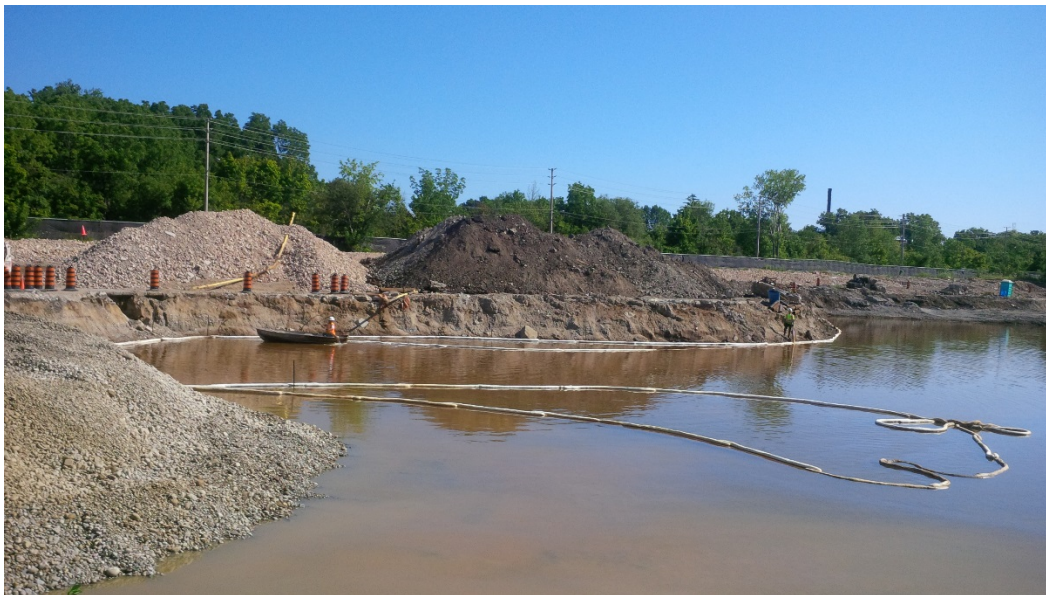
Photo 1. Boom and Skimming Operations in Wet Excavation in Contaminated Soils
