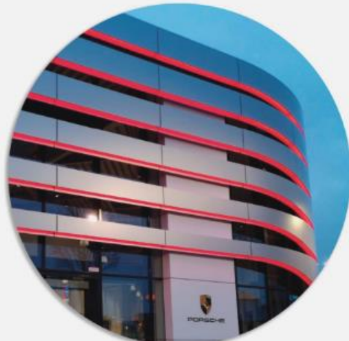
Showroom Facade E 04
