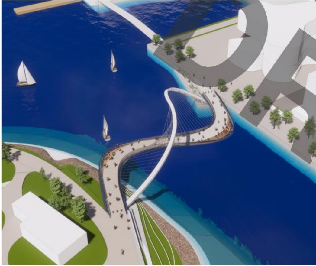
Bridge Deck Geometry and Anti-funicular Arch selected for development in final design (Competition Stage Image)
