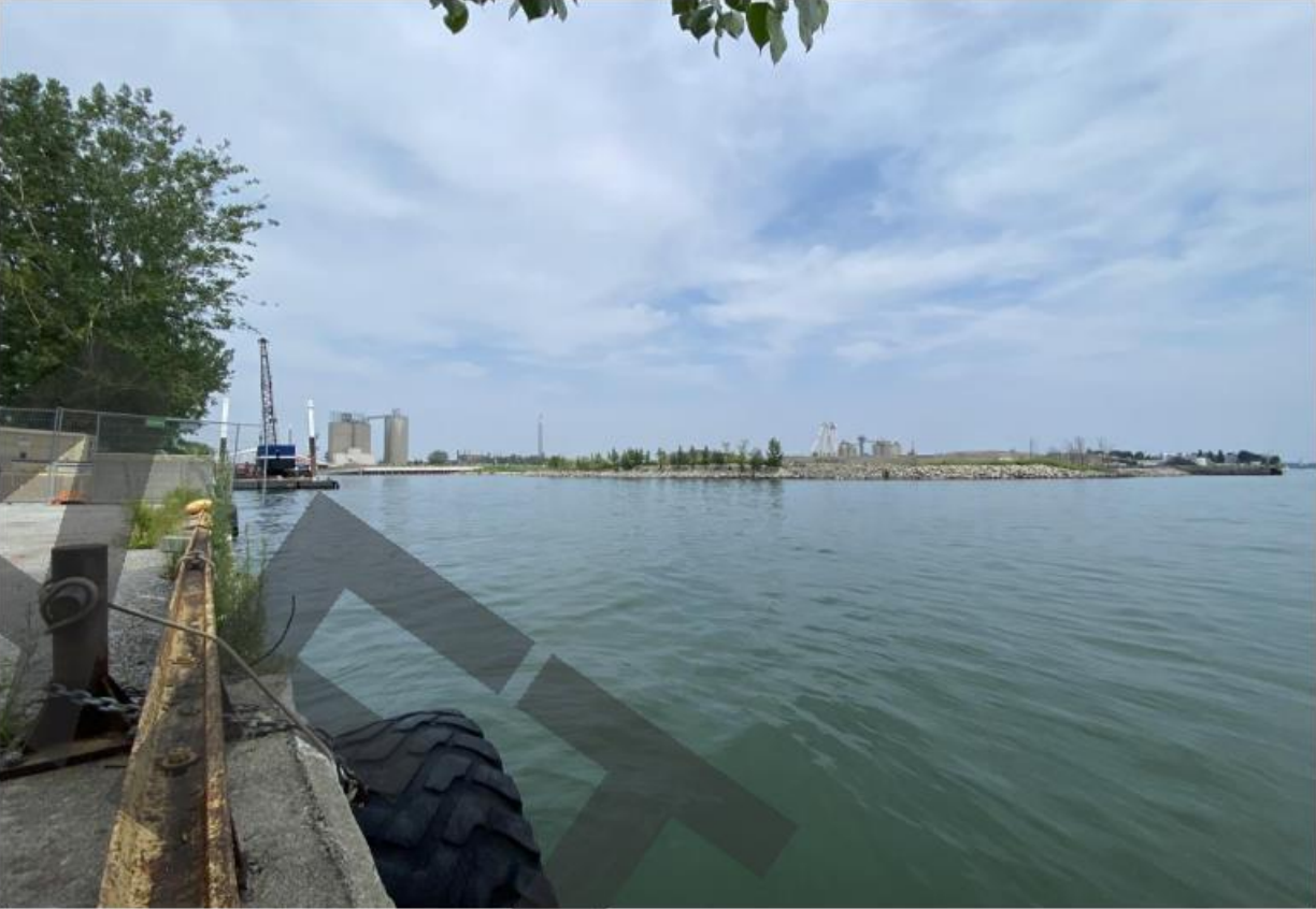
Existing site condition along the north bank with concrete slab.
