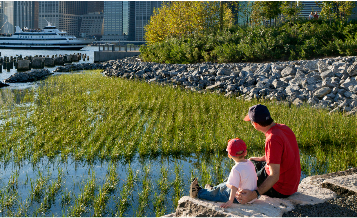
Figure 17b Example of Exposed Armour with Wetland Habitat
