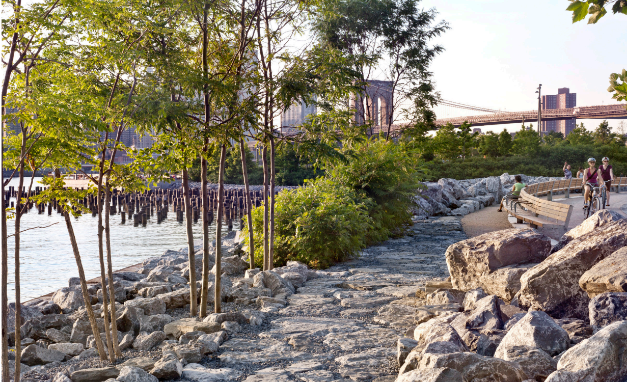
Figure 17a Example of Exposed Armour - boulders and large cobbles are used in critical areas to resist erosion from flood events and provide access to the river's edge.
