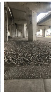
Reference Image: Yonge Street, Stabilized pebble edge adjacent to pedestrian waiting areas at medians
