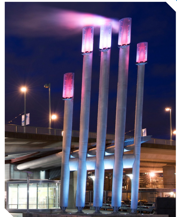
Vancouver's neighbourhood energy utility hides under a bridge and has elements that change colour with energy use. (Francl Architecture)
