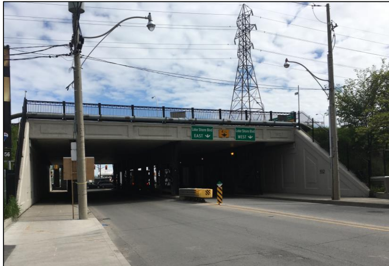
Existing structure - North side
