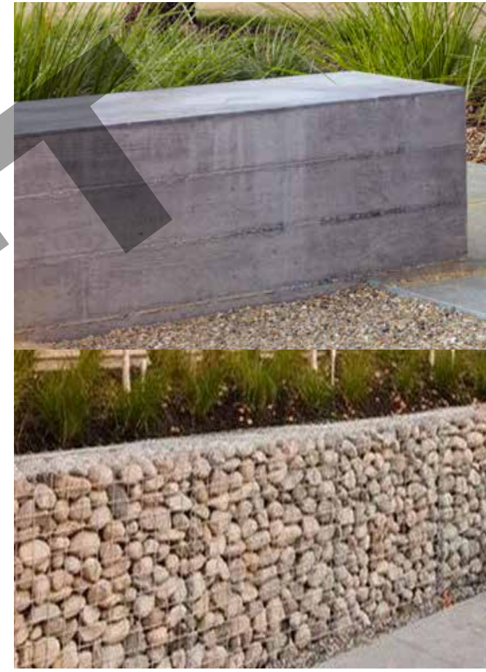
concrete retaining walls/gabion
