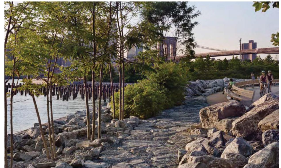
Figure A.3: Example of Exposed Armour
