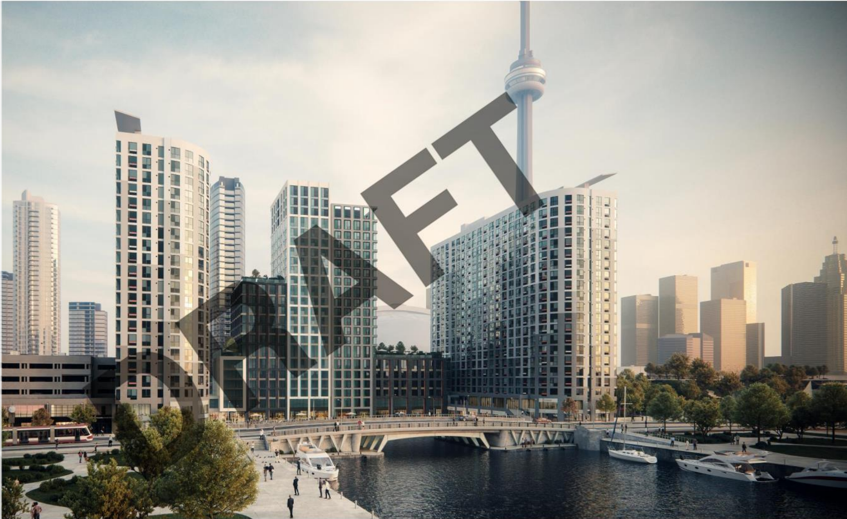
WTDRP 2 / View from Southwest
