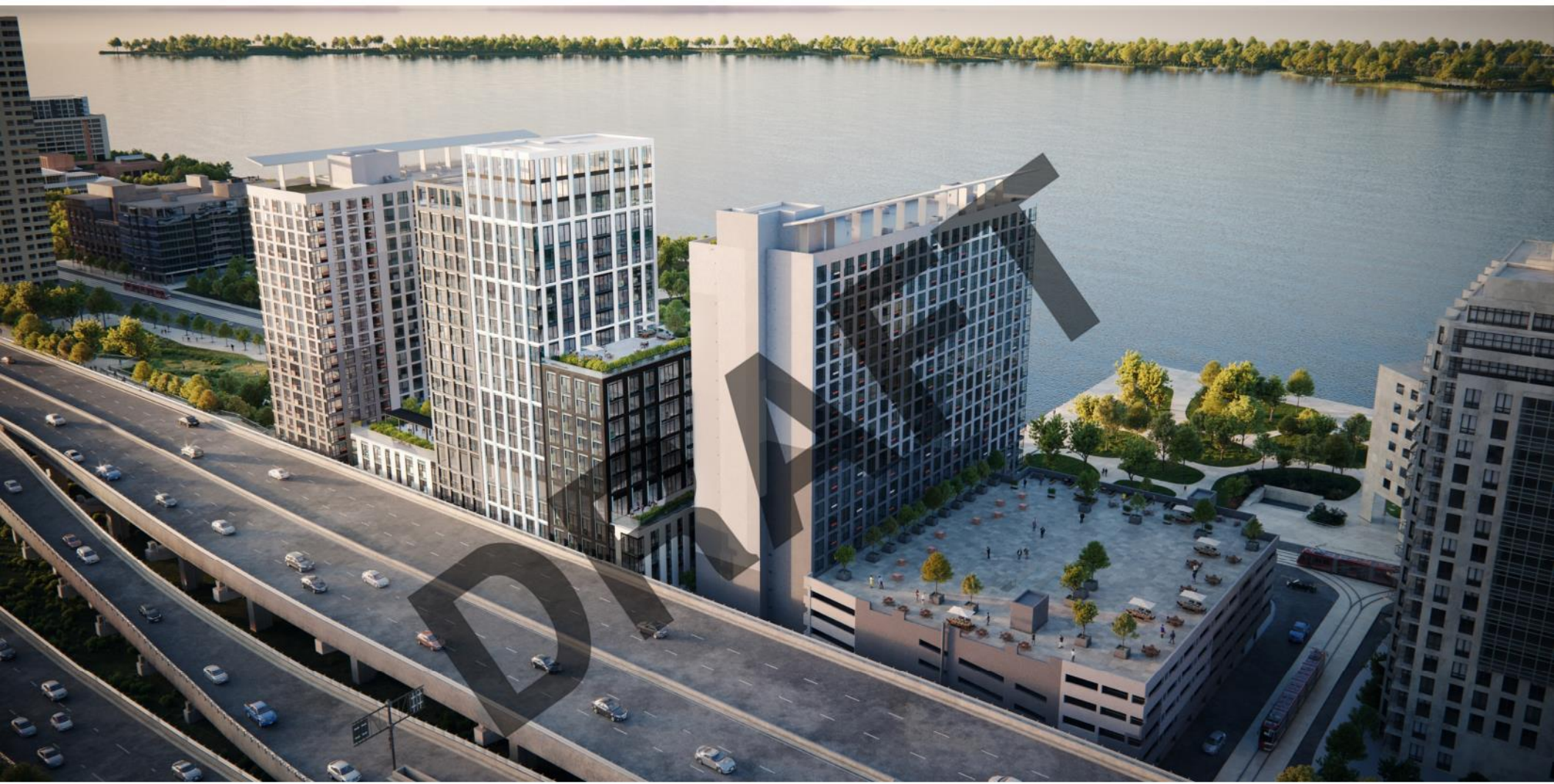
Aerial View from Northwest
