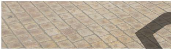
Existing Granite Sett Pavers
