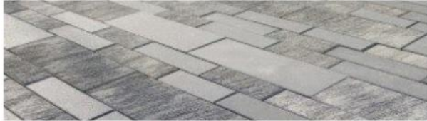
Unit Paving - Vehicular Clearway
