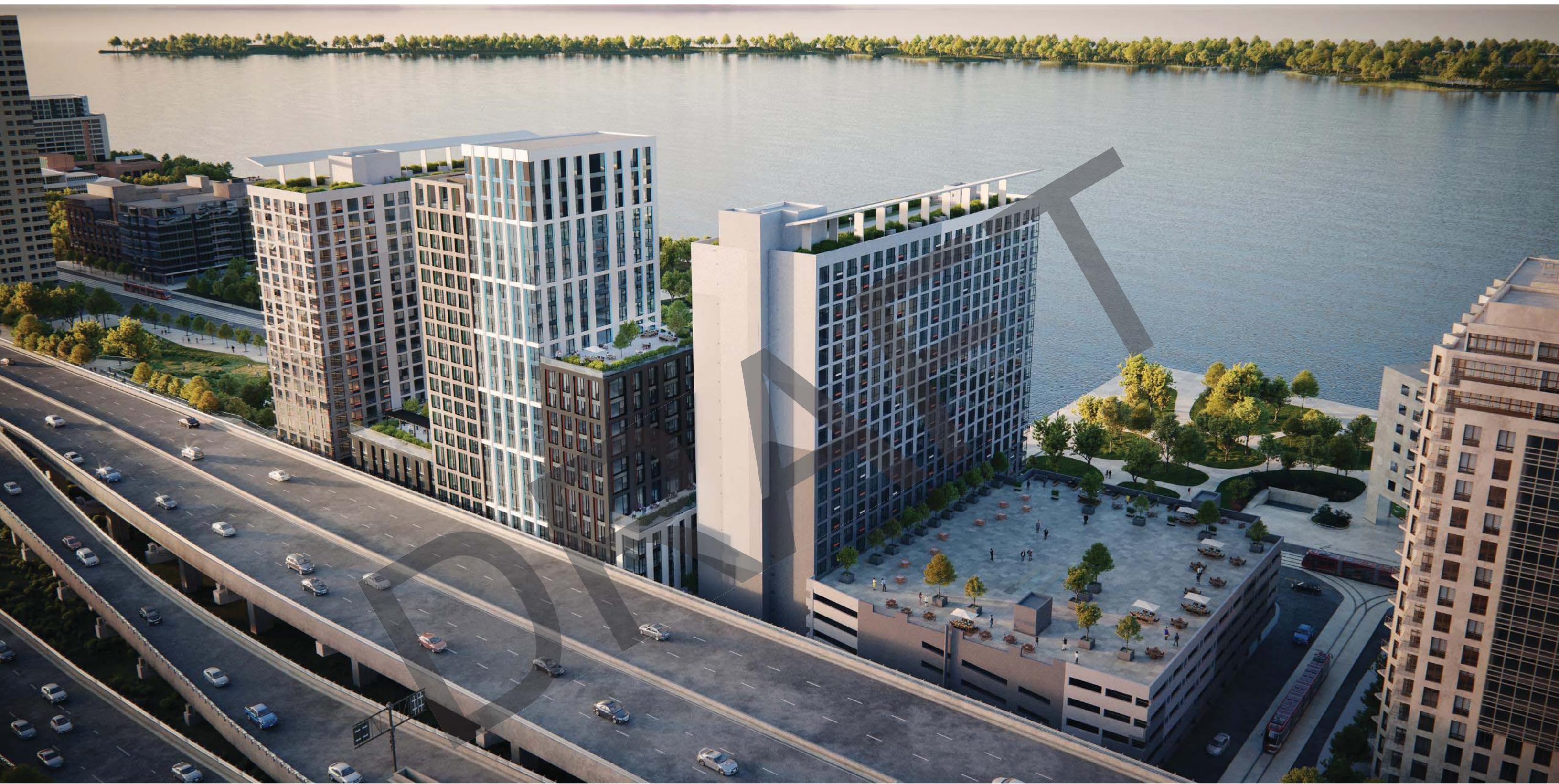
Aerial View from Northwest
