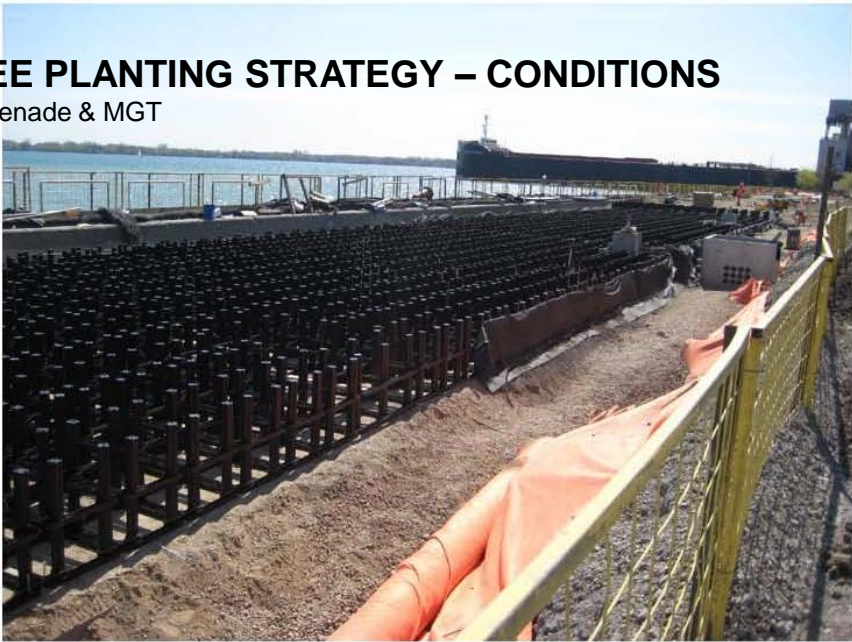
2 layers of silva Cells over granular base
