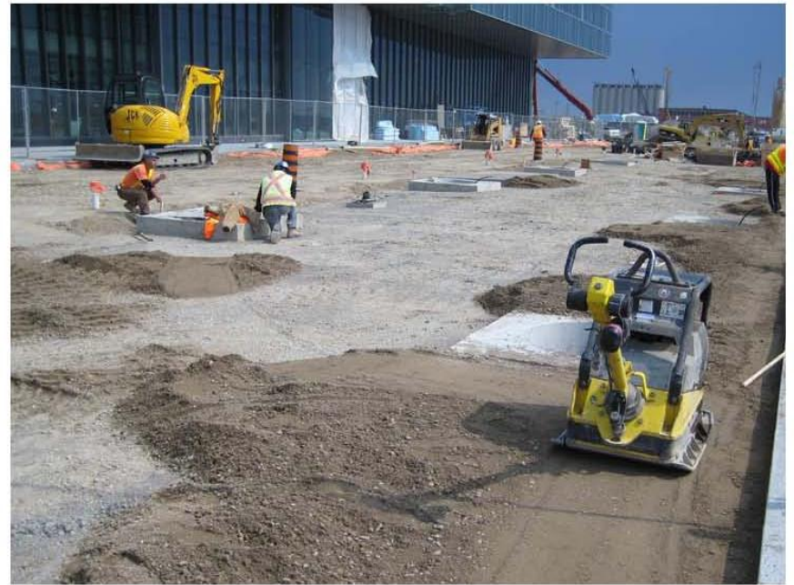
Granular over Silva Cells
