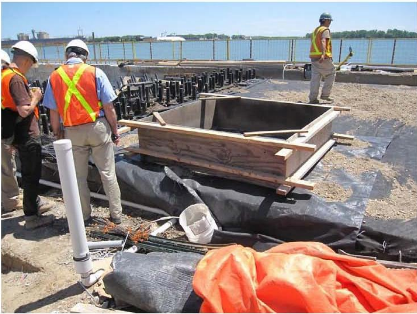
Formwork for tree pit over Silva Cells
