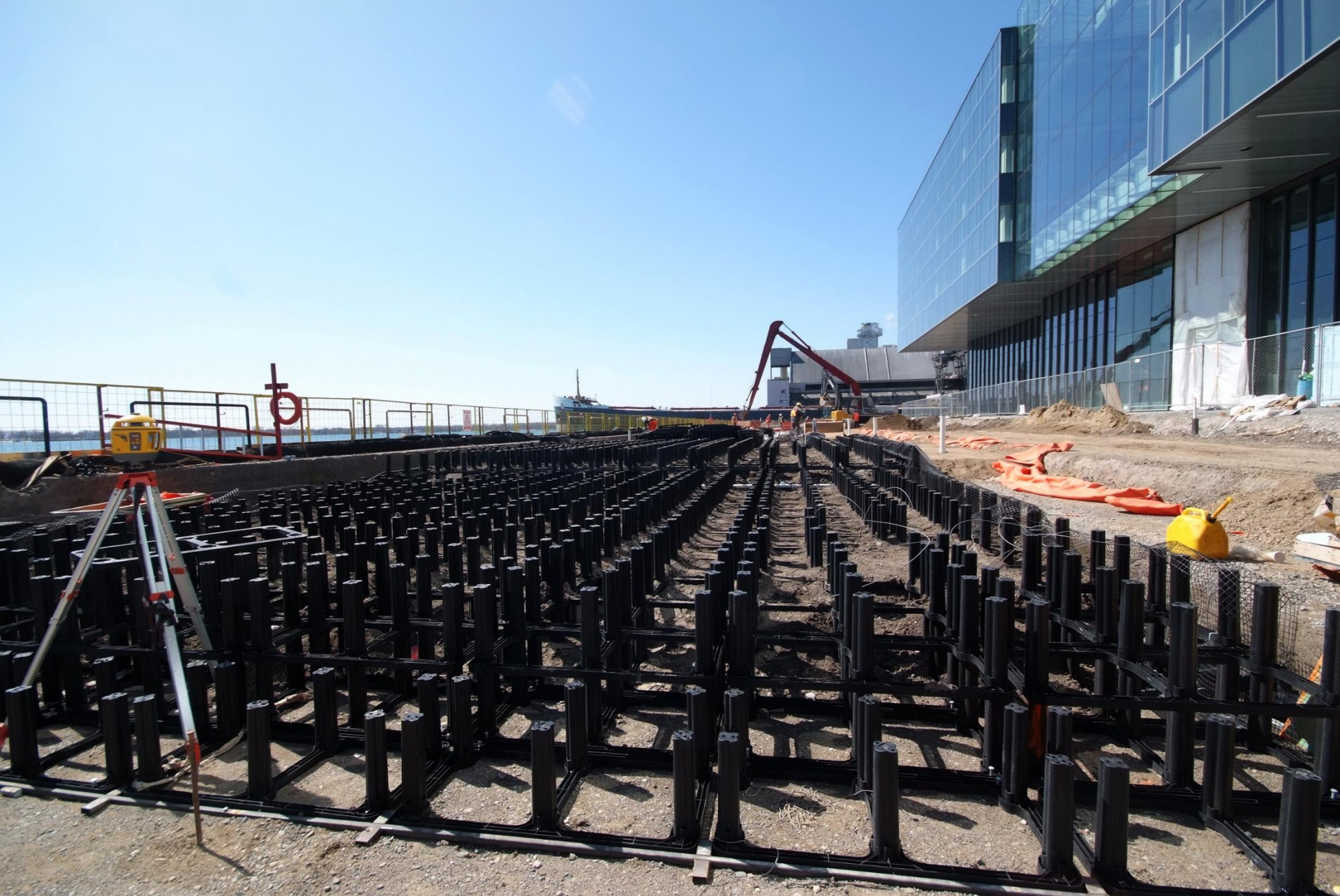
Silva Cell Installation
