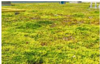
SEDUM EXTENSIVE GREEN ROOF
