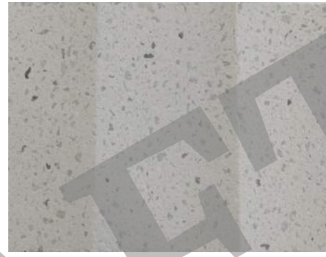
TOWER - 8A / 8B SANDBLASTED PRECAST CONCRETE
