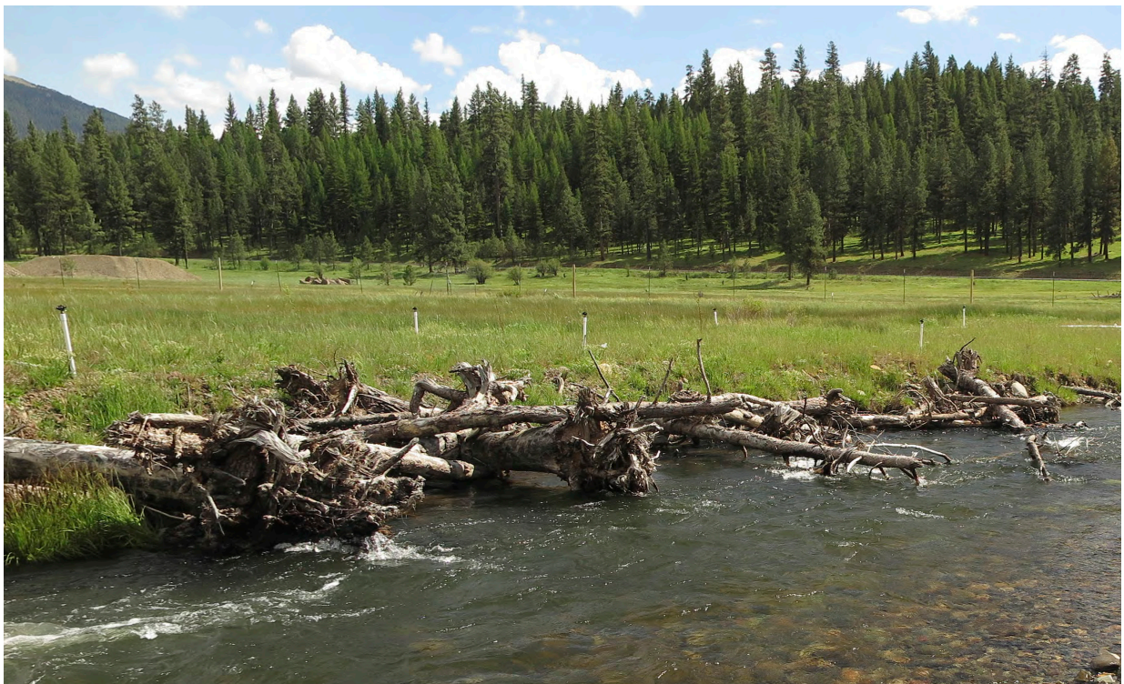
Figure 19 Example of Large Wood Stabilization - large wood installed in the bank toe provides erosion resistance, as well as excellent aquatic and terrestrial habitat.
