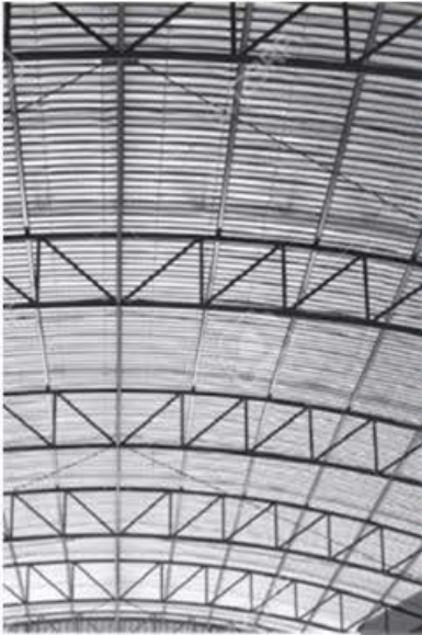
ENGINEERED STEEL TRUSS ROOF STRUCTURE
