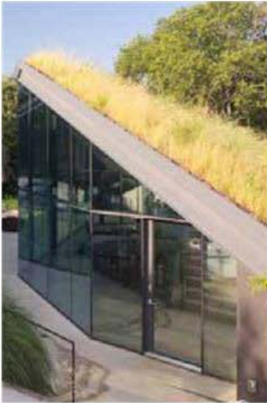
VEGETATED GREEN ROOF
