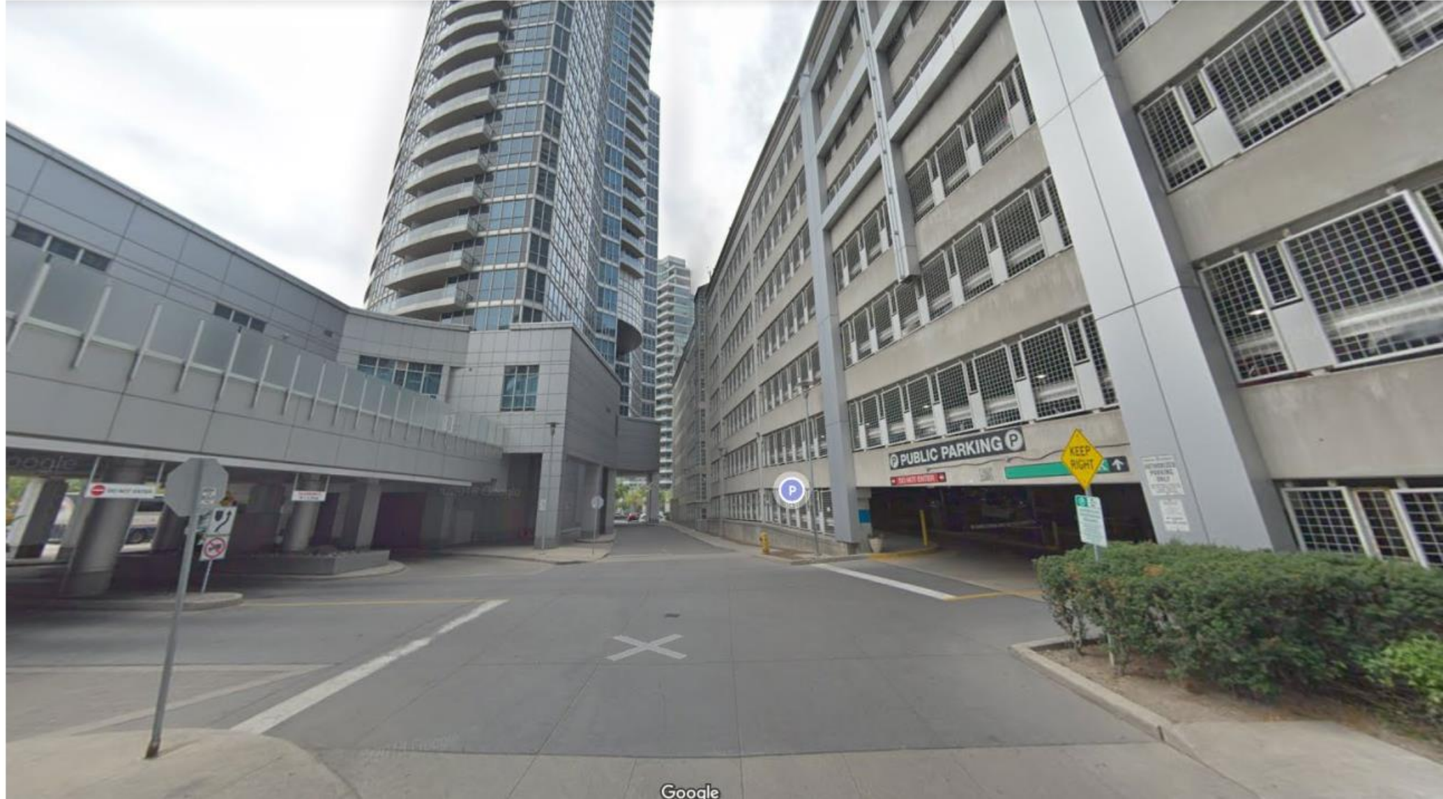
Entrance to existing parking structure from the Waterclub Condos
