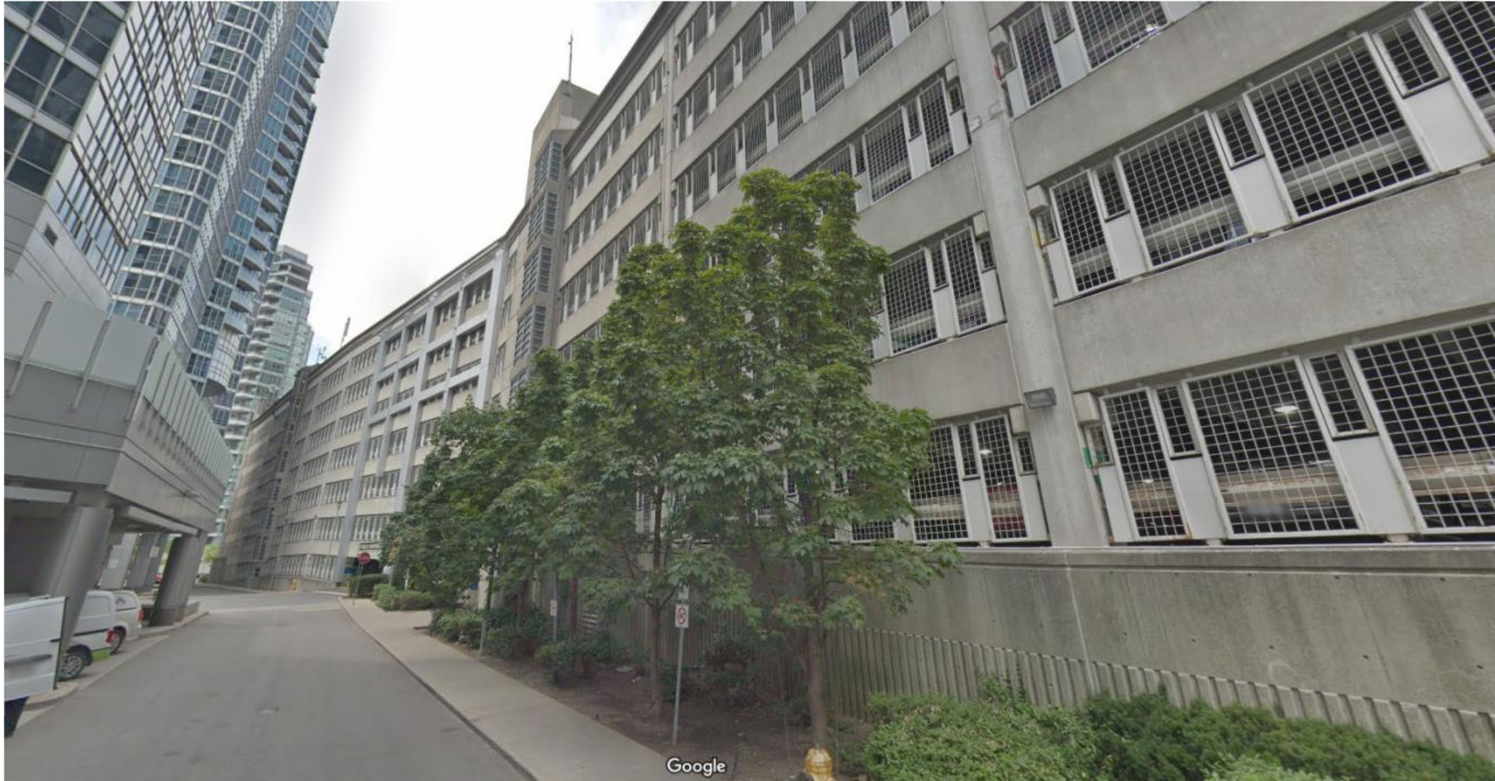
South elevation of existing parking structure from the east end of the laneway
