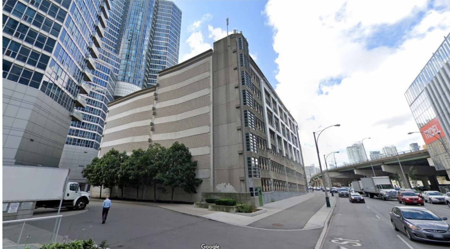
Harbour and York looking southwest
