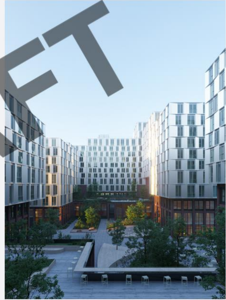
Looking west from above the amenity deck
