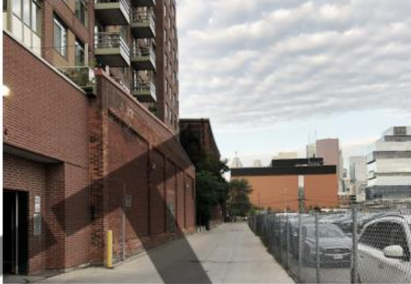
South edge of the site looking West
