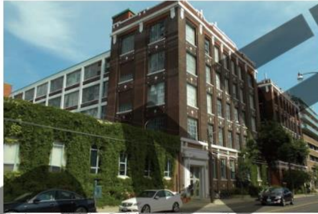
Carlaw at Wrigley Building, facing southeast.
