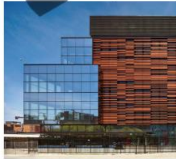
Equinix Data Centre, Toronto
