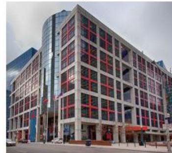
CBC Broadcast Centre, Toronto
