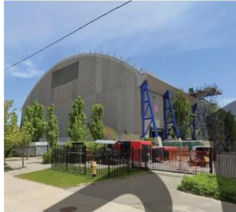
Pinewood Mega Studio (Alsop)
