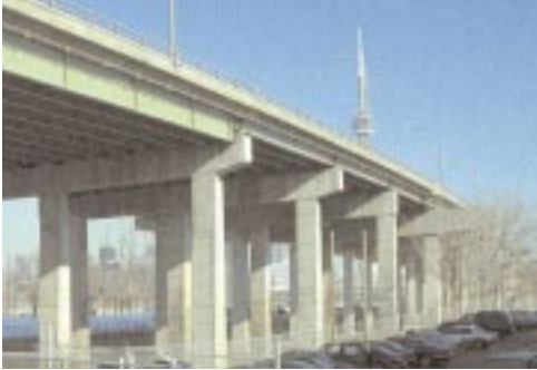
View of Gardiner at Fort York
