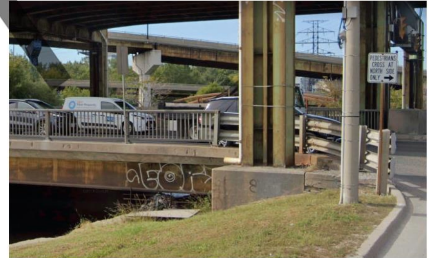
Existing Condition - Bridge and Bent at Intersection
