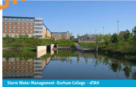
Storm Water Management -Durham College - dTAH
