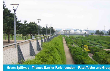
Green Spillway - Thames Barrier Park - London - Patel Taylor and Groupe
