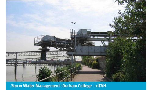
Storm Water Management -Durham College - dTAH
