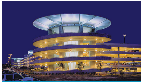
Raleigh Durham Airport Parking Structure - The Freelon Group
