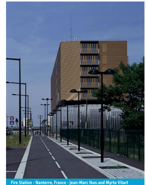
Fire Station - Nanterre, France - Jean-Marc Ibos and Myrto Vitart
