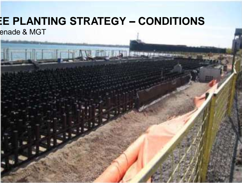
2 layers of Silva Cells over granular base
