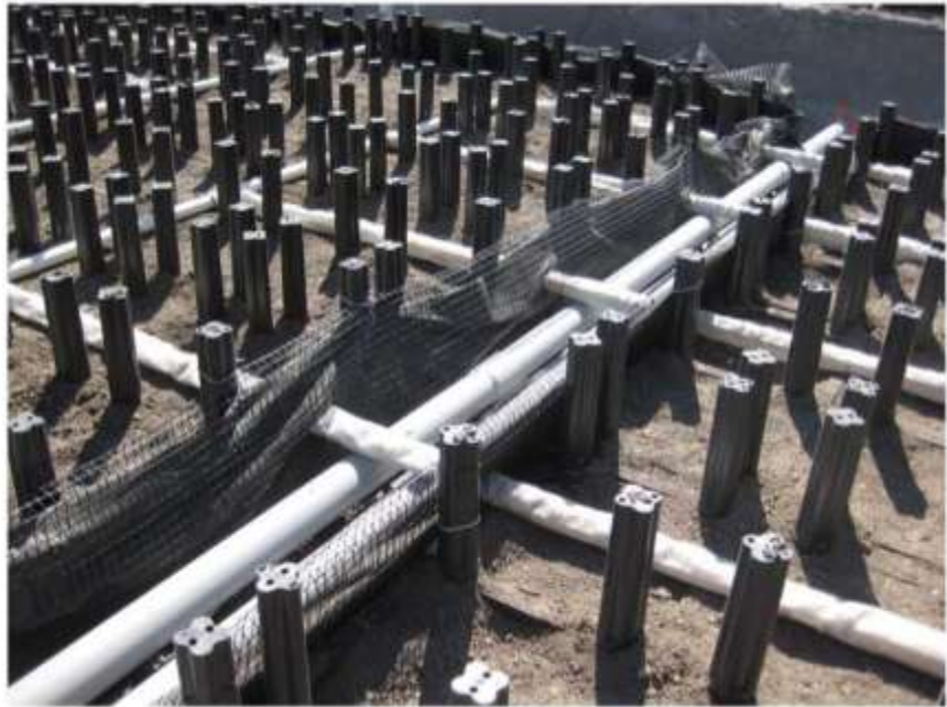
Electrical ducts and Irrigation through Silva Cells
