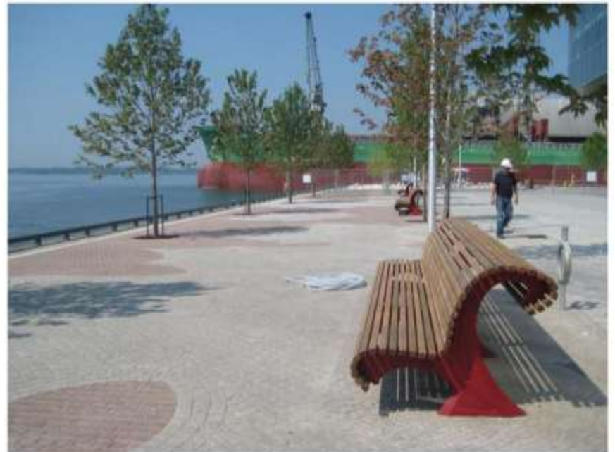
Finished surface over Silva Cells
