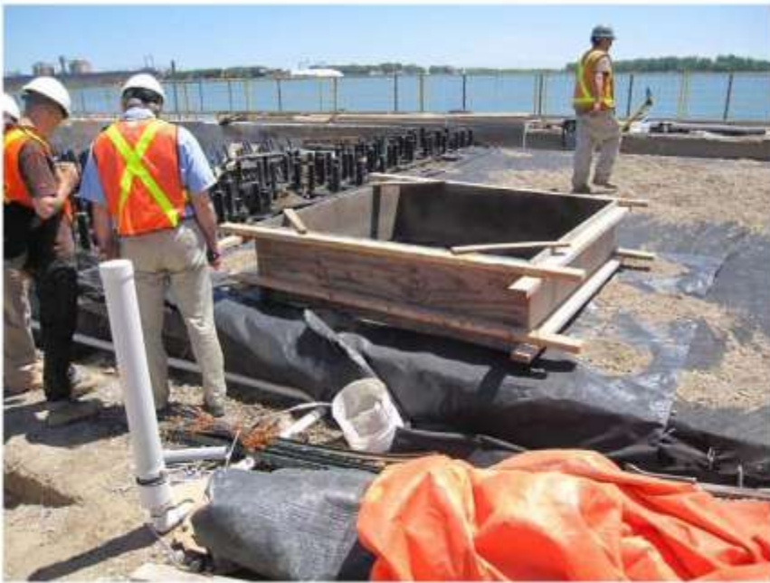
Formwork for tree pit over Silva Cells
