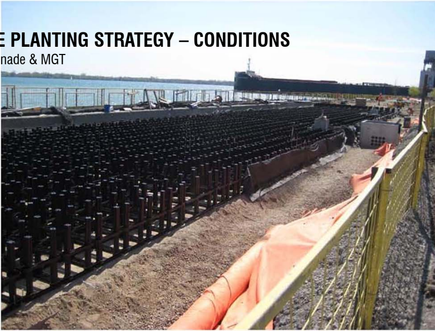
2 layers of Silva Cells over granular base
