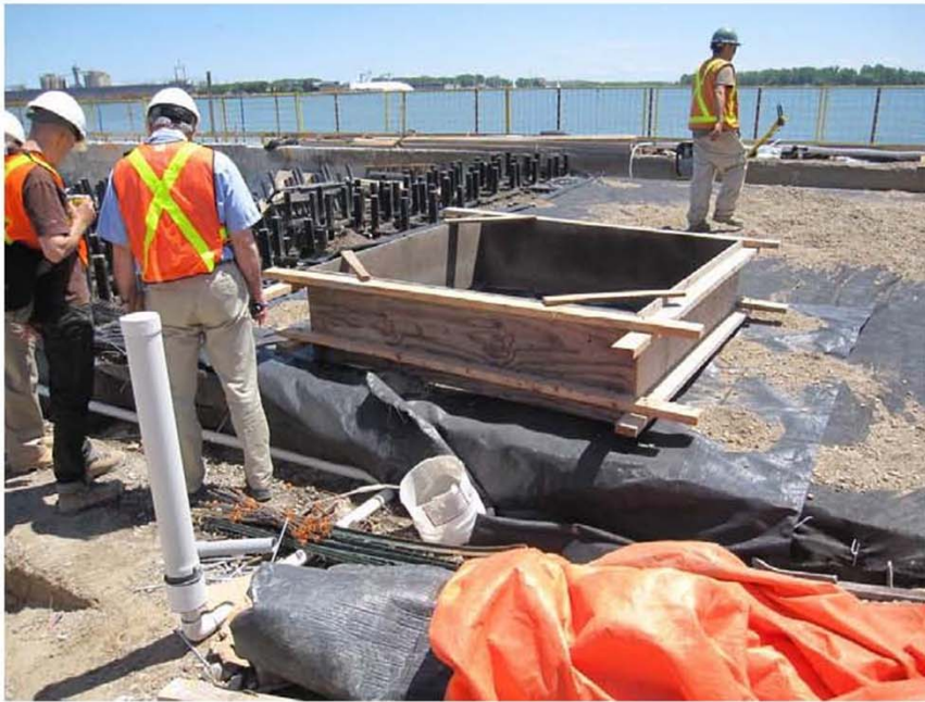
Formwork for tree pit over Silva Cells
