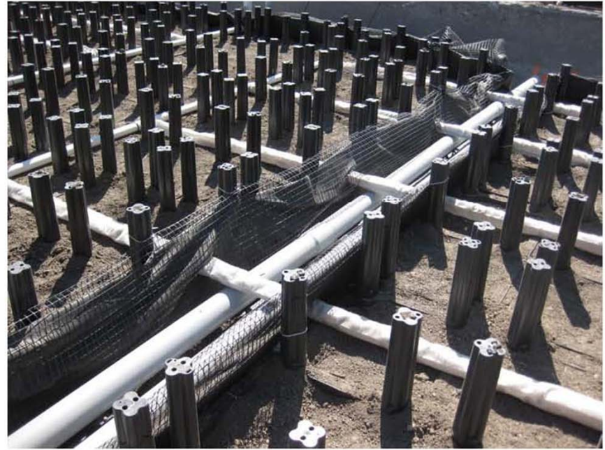
Electrical ducts and Irrigation through Silva Cells
