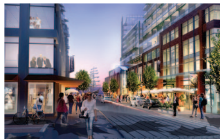
A significant retail and entertainment destination on Bonnycastle Street will draw visitors from across the city and will provide connections to neighbouring public spaces, including Sherbourne Common, Queens Quay linear park, and the Water’s Edge Promenade.
