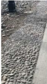
Stabilized stone as median edge
