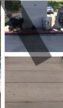
CIP Concrete w/special saw cuts and finish
