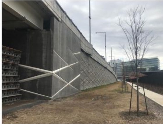
Montreal Bonaventure Expressway at Lachine Canal Retaining wall and underpass patterned concrete
