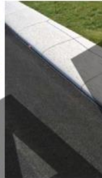
Asphalt with Concrete Soft Curb
