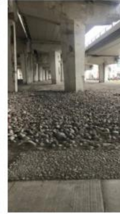
Reference Image: Yonge Street, Stabilized pebble edge adjacent to pedestrian waiting areas at medians
