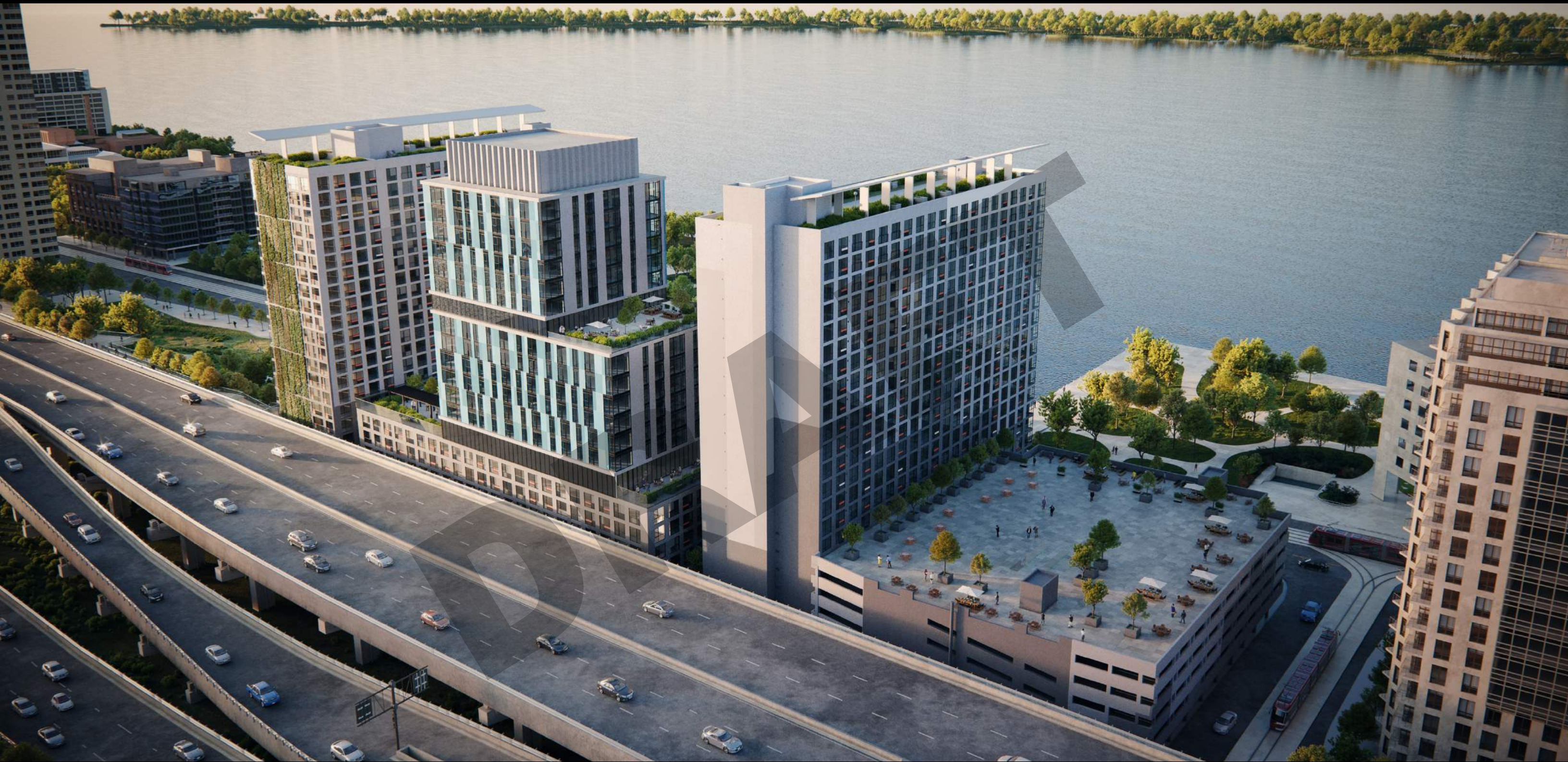
Aerial View from Northwest
