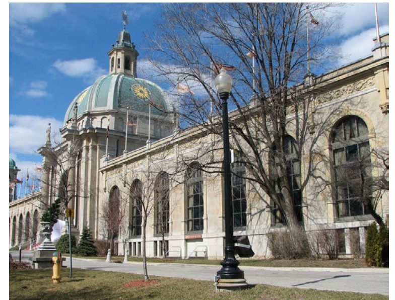
CNE ONTARIO GOVERNMENT BUILDING BEAUX-ARTS ARCH.
