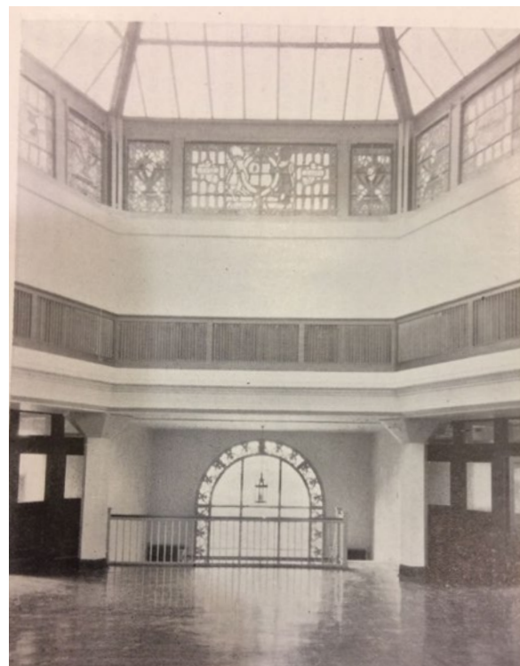
INTERIOR OF THE HEXAGONAL PAVILION IN 1927
