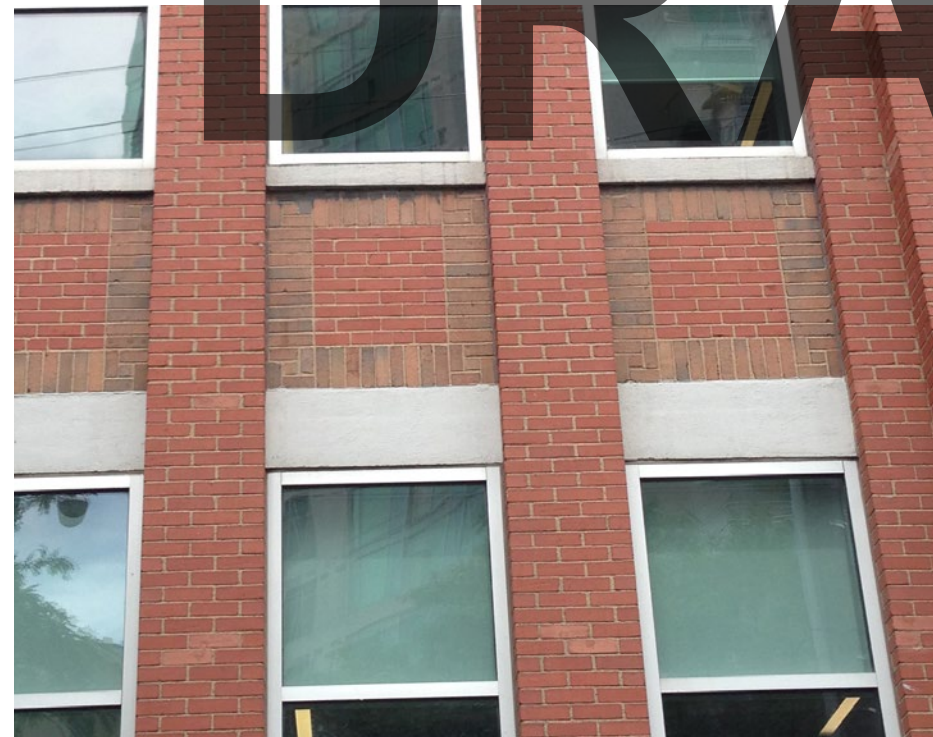
BLDG'S EXTERIOR DETAILING INCLUDING RED BRICK MASONRY, PRECAST STONE SILLS & LINTELS
