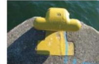
Preserve existing mooring elements where possible - paint anthracite grey (RAL 7016)
