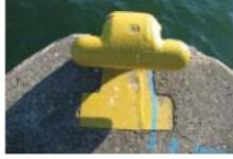
Preserve existing mooring elements where possible - paint anthracite grey (RAL 7016)
