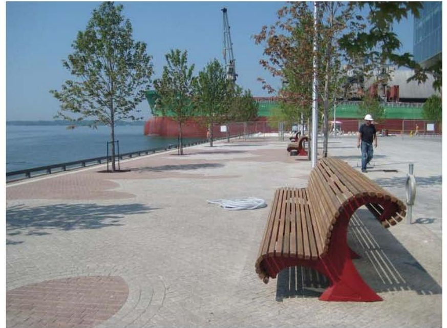
Finished surface over Silva Cells
