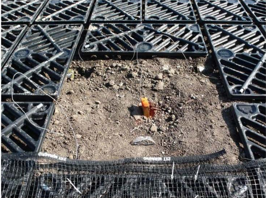
Tree pit opening in top deck of Silva Cells
