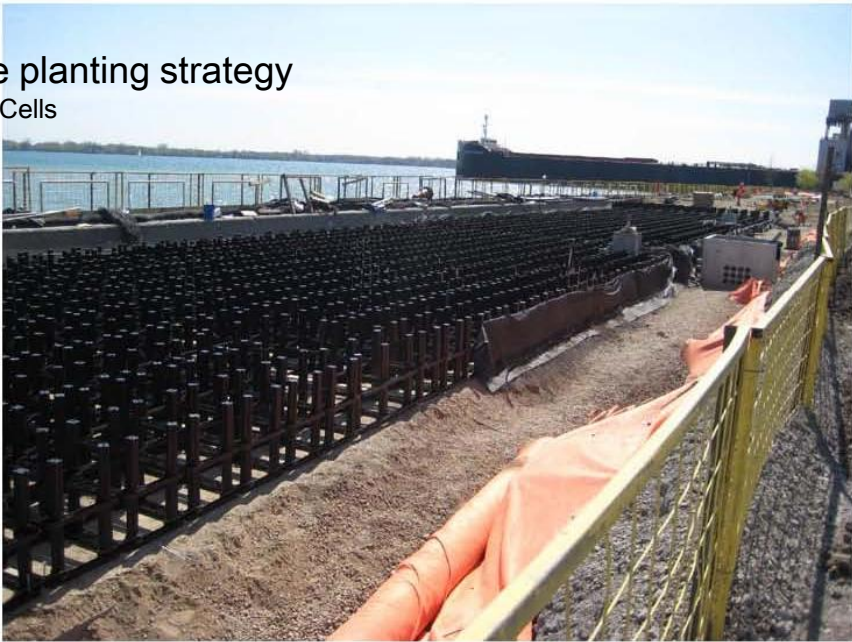
2 layers of silva Cells over granular base
