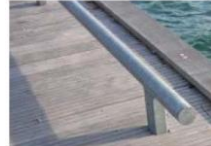
Galvanized steel toe rail
